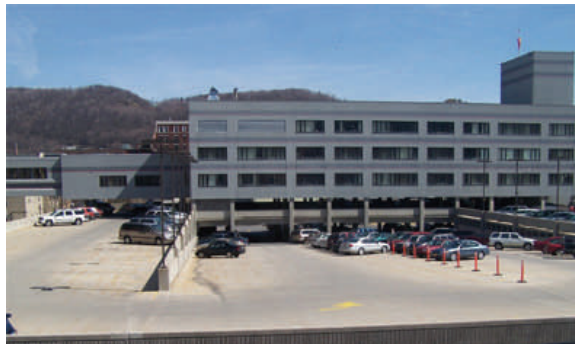
Seifert Parking Garage, also known as the Main Street West Parking Garage.
